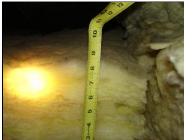
8" of fiberglass = aprox 24 R Value -32 min
